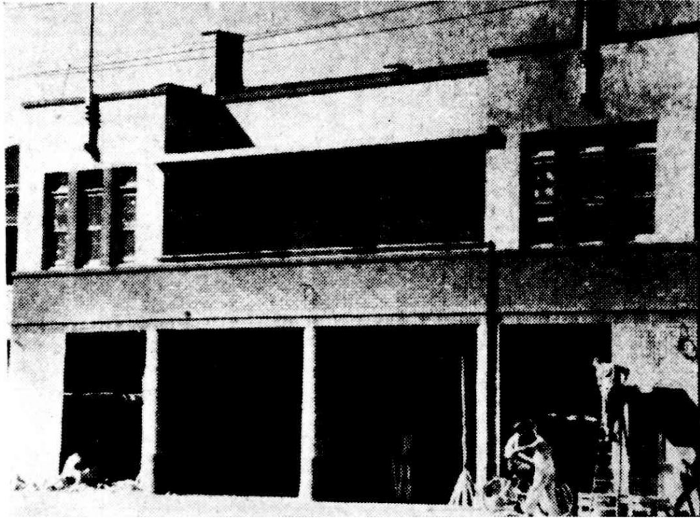
RIGHT—With scaffolding removed, the lines of the remodelled fire brigade headquarters, Wakefield street, can now be seen.
